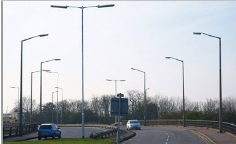
Figure 7: Example of street light profiles to be avoided where possible
